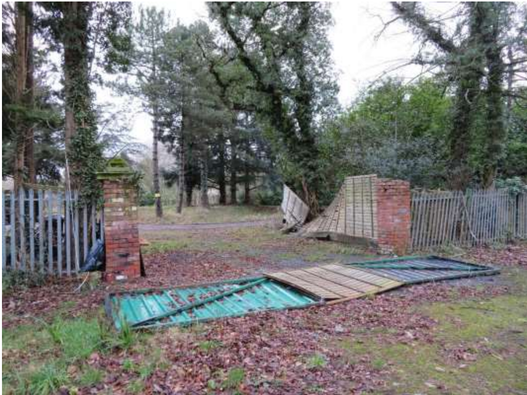
Plate 10 The private gateway created by Samuel or William Cunliffe Brooks to lead onto Brooks Drive. It is currently in poor condition.
